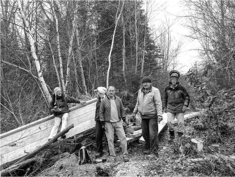
Recovering Foot-Bridge After Flood
